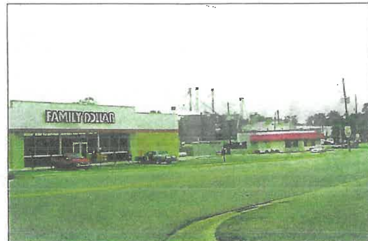
Auto-Oriented Commercial Uses along NC 581, Bailey NC
